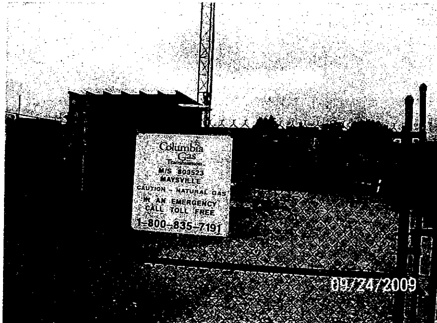
The natural gas service is provided by Columbia Gas. www.columbiagasky.com Columbia Gas transmission station entrance access.
