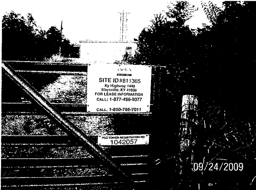
Radio tower entrance access
